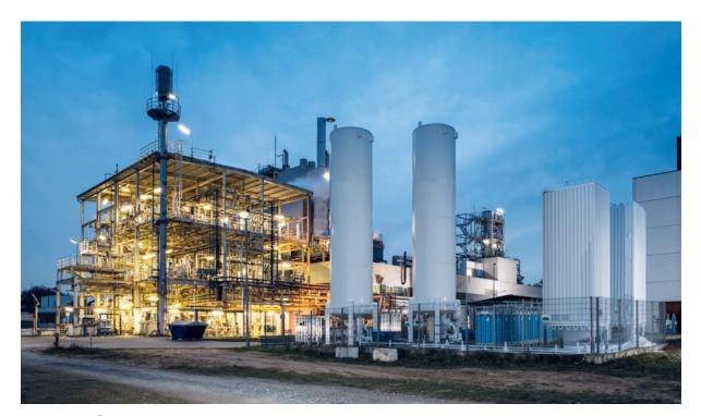
Figure 4: bioliq<sup>®</sup> plant at the Karlsruhe Institute of Technology for the production of BTL (biomass-to-liquid) fuels via synthesis gas, DME and OME. (© KIT)
